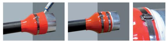
**3.** Inject the adhesive included in the delivery all round underneath the sleeve. Then install the second strap. Spread leaking adhesive, if necessary.
