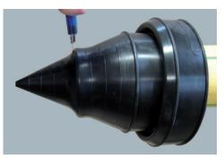
2. Cut off sleeve in front of the carrier pipe with a sharp knife. Then pull sleeve over the carrier pipe up to the casing pipe (sleeve can be stretched about 10 %).
