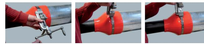
3. When reaching maximum stress, slowly bend over the strap about half a turn while releasing the crank.
